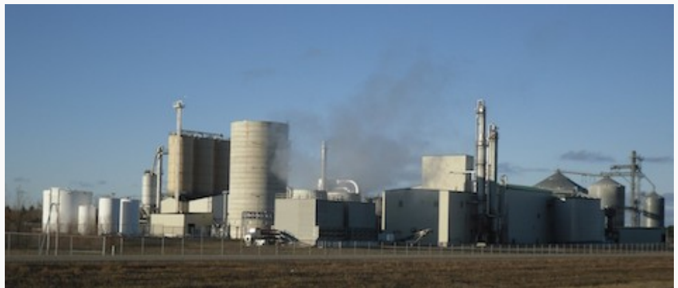
The CMEC 23 million gallon per year ethanol plant in Little Falls, Minnesota.
